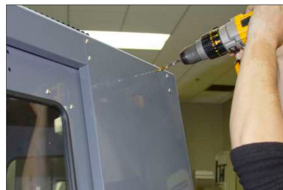
Figure 4-169: Drilling holes into the top of the enclosure.
