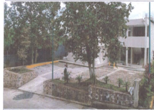
F5: Fachada principal
