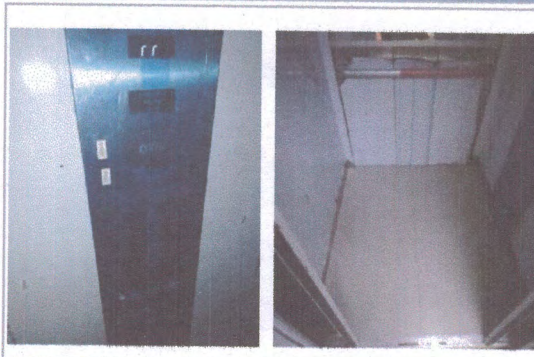
F4: TABLERO PRINCIPAL
