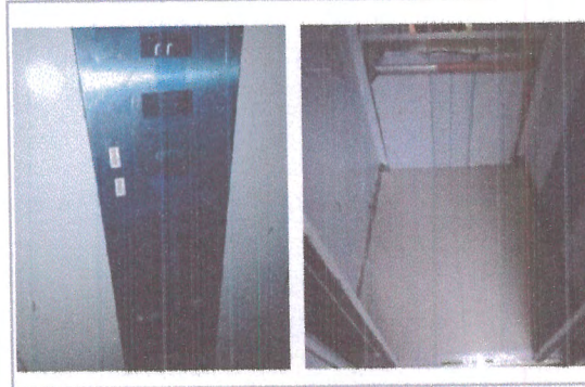
F4: TABLERO PRINCIPAL
