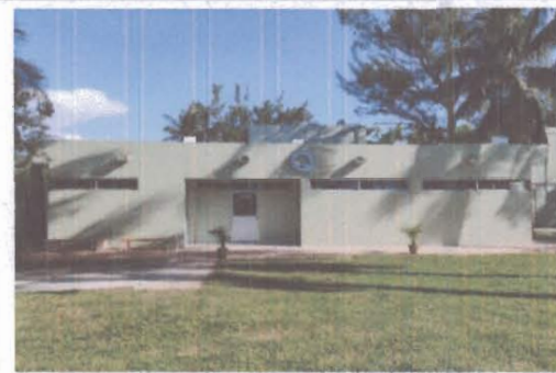
F2: Fachada principal
