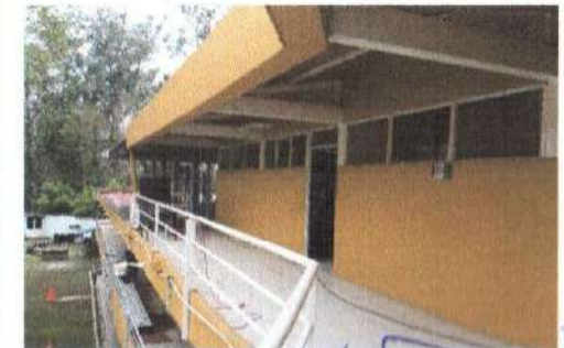
F5: Vista exterior
