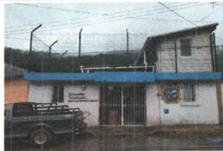
F4: Fachada principal
