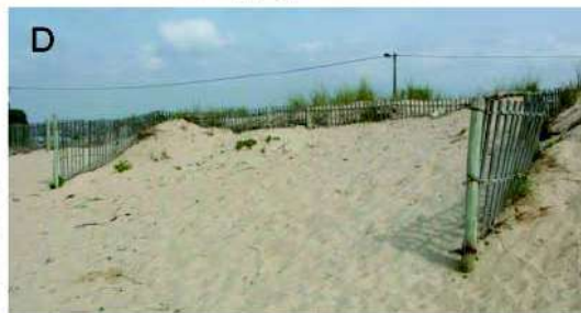
A sand fence system filled with sand and highly ineffective
