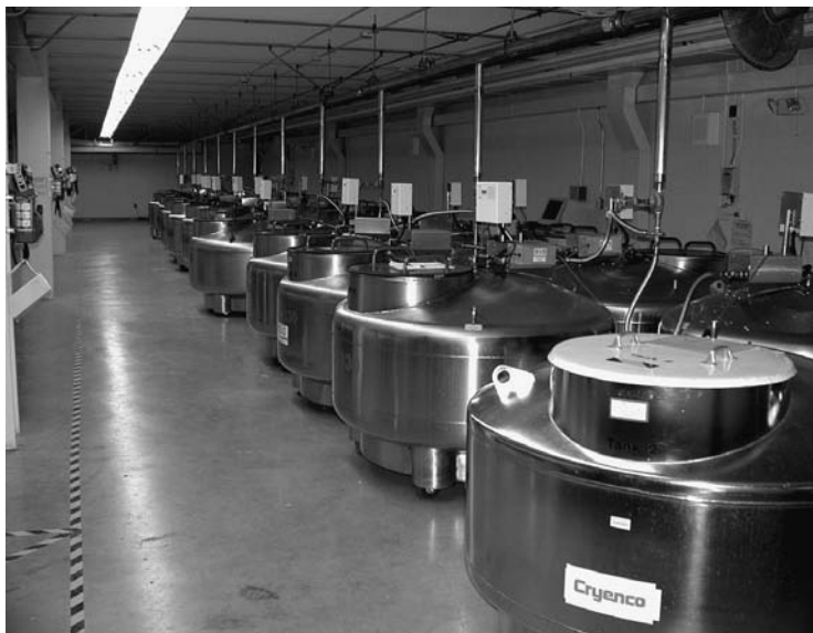
Fig. 17.3. The cryopreservation tanks for storing vegetative plant tissues at -196^{\circ}\text{C} in liquid nitrogen and for seed at -160^{\circ}\text{C} in liquid nitrogen vapour phase at the National Center for Genetic Resources Preservation, Fort Collins, Colorado, USA.
